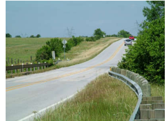
Pre-existing FM 1171 before widening
