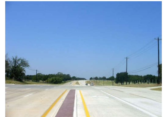
Existing FM 1171 after widening
